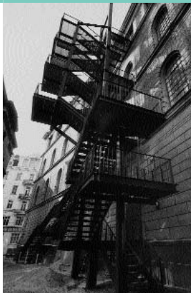
Fire Escape on the north wall
