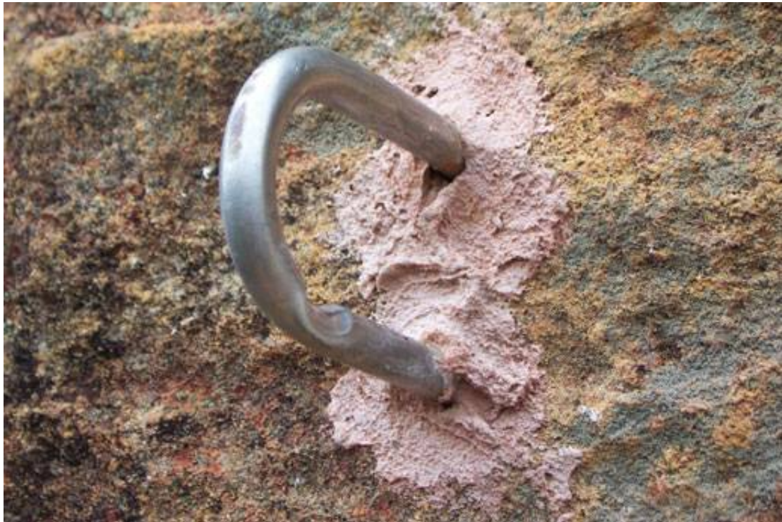
Figure 5 Badly placed Ubolt showing major wear after 4.5 years service
